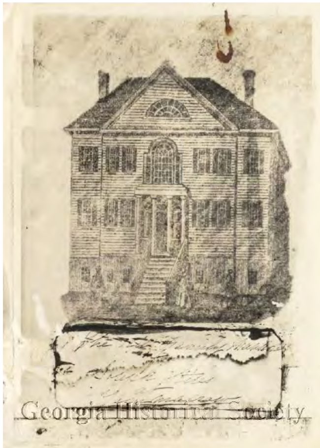
Figure 3: Clay-Stiles House which sat near the present day intersection of Bay and Fahm Streets. (Georgia Historical Society).
