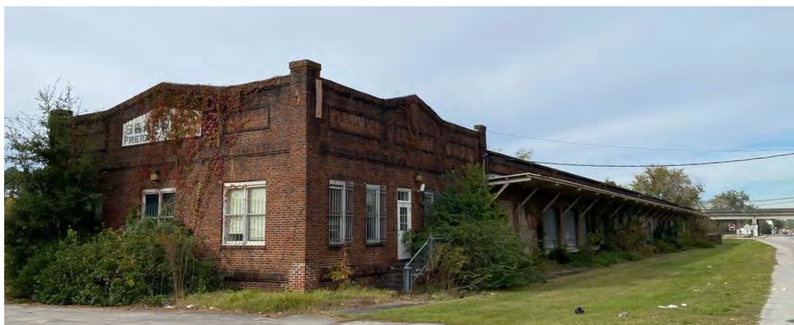
Figure 58: Seaboard Freight Station at 703 Louisville Road, built 1929 (Ethos).
