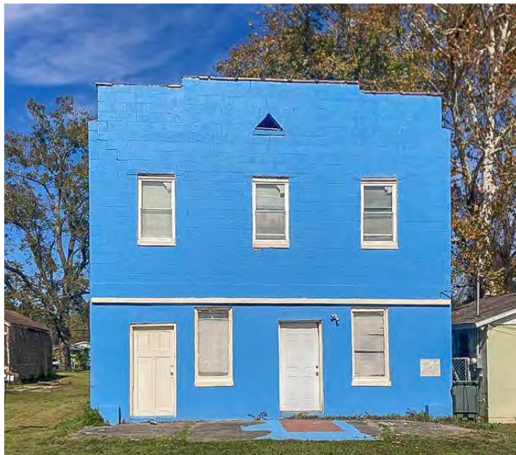
Figure 62: Commercial Building at 1416 W Gwinnett Street built circa 1940 (Ethos).
